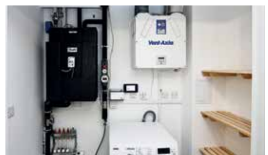
□ An apartment utility room
