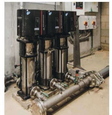
□ Basement cold water booster set
